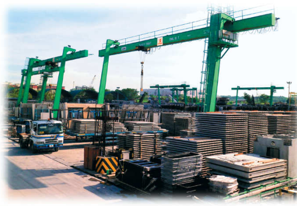
Precast Yard in Singapore
